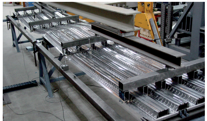
Figure 9 Continuous decking tests at the construction stage
