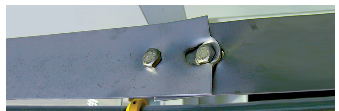
Figure 11 Failure of bolted specimen by block tearing and net section failure mode
