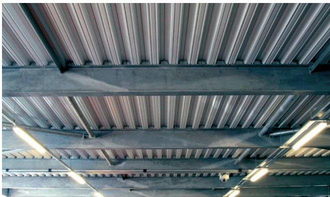
Figure 8 Composite floor with exposed soffit in a car park
