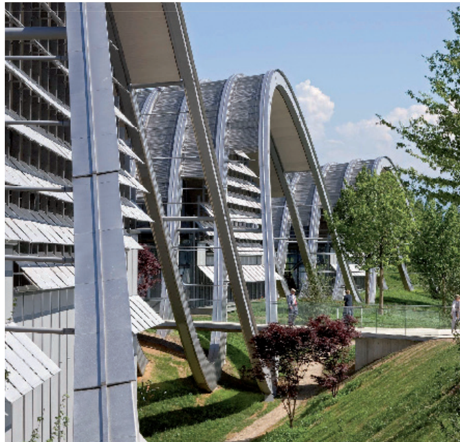
entrum Paul Klee, Suisse Renzo Piano Building workshop In collaboration with ARB (Bern) © RPBW – Michel Denancé Achieved with grades 304, 316L Uginox Top finish
